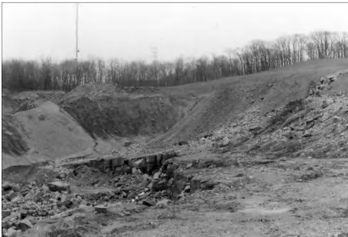
Figure 6. View of Jesse Pit looking north. Working face in quartzite in foreground; sand and gravel face behind. Slope in background near tree line is reclaimed pit area ready to be seeded.
