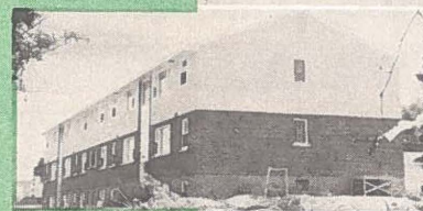
The new Dagsrik Apartment House.
