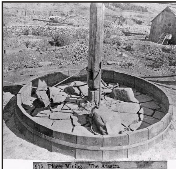
Figure 7. An arastra from the U.S. midwest, circa. 1890's. Image from http://www.calisphere.universityofcalifornia.edu/
