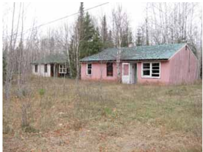
Photo 18. Abandoned houses in former town site of Burchell Lake.
