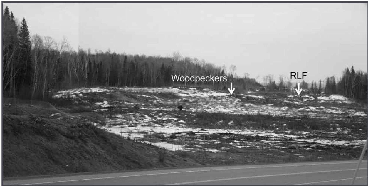
Figure 19 View northeast from existing highway along the construction zone. Note the ‘bank’ in the clearing (left side of frame) that likely is the former Lake Minong strandline. In the foreground the current highway cuts through this former beach feature. Note the location of the Woodpecker I, II, and RLF sites along the beach strand line. The former is located on the northwest side of a bedrock knob, while the RLF site is a small flaking station located on a berm (perhaps a high storm beach) overlooking the main strand line.
