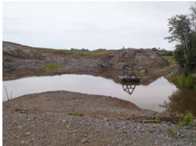
Photo 5. Storm water collection pond. Pump barge can be seen in centre of pond. Water is pumped to tailings pond at Dam No. 4.
