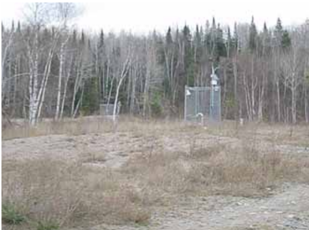
Photo 17. No. 4 Shaft and 250 Vent Raise are located below fenced vent pipes. Fencing was installed to protect against vandalism.
