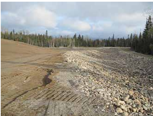
Photo 14. Reconstructed eastern perimeter spillway. East side of tailings relocation area can be seen to left.
