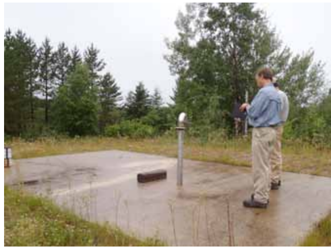
Photo 1. Reinforced concrete cap, Shaft No. 1 - Discovery Point
