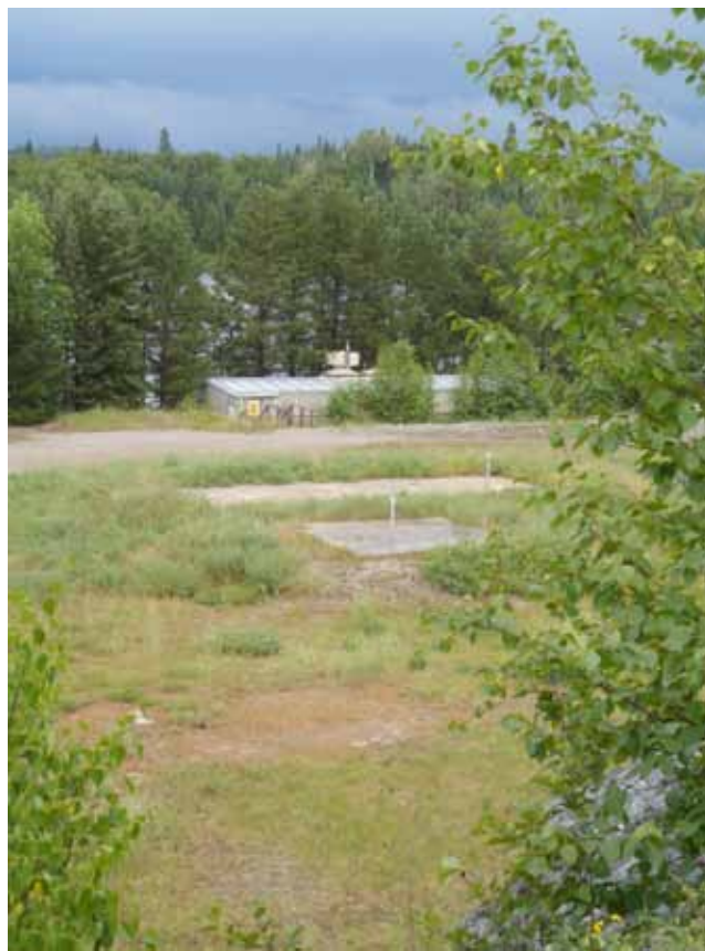
Photo 3. View of No. 2 Shaft area. Concrete caps and pump house are visible in centre of photo.
