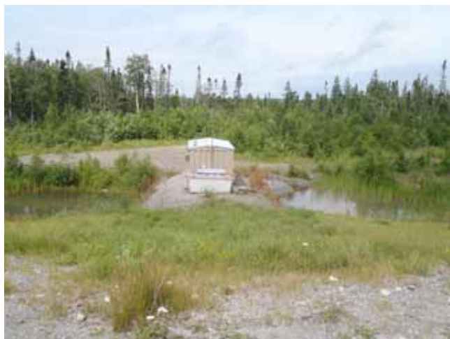
Photo 7. Dam No. 4 seepage collection pond and pump house
