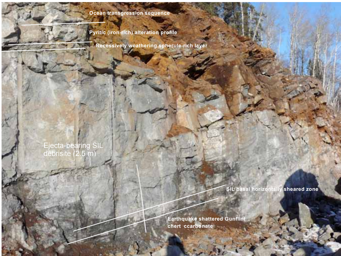
Figure 11. The current Terry Fox outcrop is a nearly featureless gray carbonate face. Given several decades of weathering, faint features within the debrisite should begin to appear as in Figure 12. White vertical scale is 1 m. Rusty area is weathered rock.
