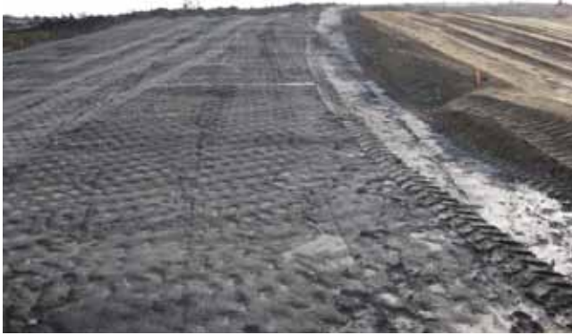
Photo 13. Photograph taken in October 2011 during placement of cover over relocated tailings at TMA-1. Clay layer is visible to left, with overlying granular cover layer to right
