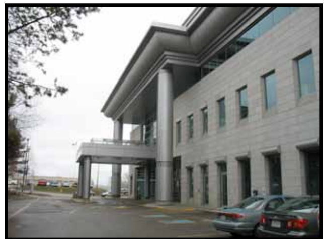
Figure 7. Entrance of the Ontario Government Building with the flame-finished Butler Grey granite on the exterior and features of the Post Modern architecture.
