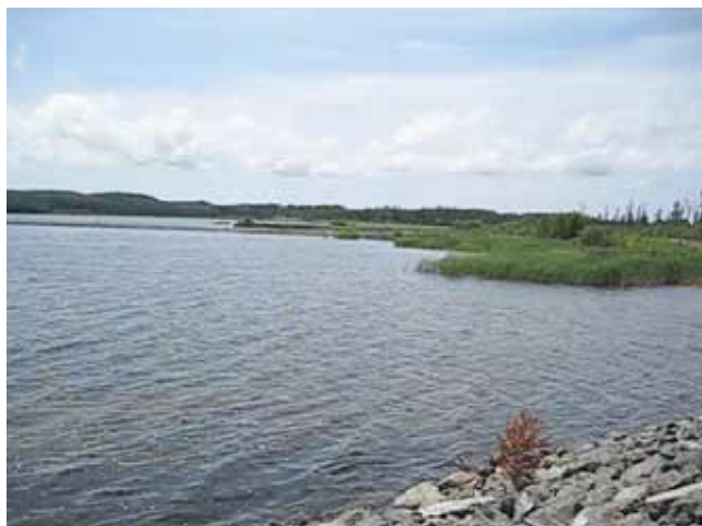
Photo 6. Shebandowan Mine tailings pond. Dam No. 4 is located to right hand side of pond. Splitter dyke can be seen at centre of photo crossing pond. This dyke limits wave development in pond.
