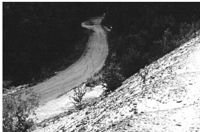
Photo 11. Embankment on west side of TMA-1 in 1998.
