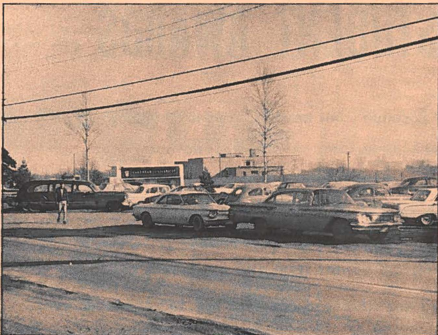
Oliver Road overflow
