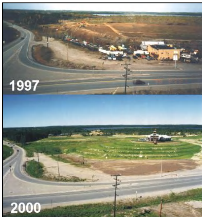
Figure 39. Pre- and post-rehabilitation views of the MacLeod-Cockshutt tailings at the junction of Highways 11 and 584, showing new Heritage Interpretative Centre.
