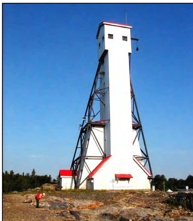
Figure 34. No. 1 Shaft headframe, MacLeod-Cockshutt Mine (Stop 2-1).
