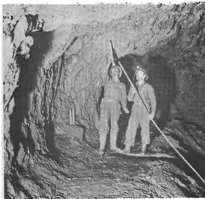
Figure 3 - Underground Sub-Level Stopping
